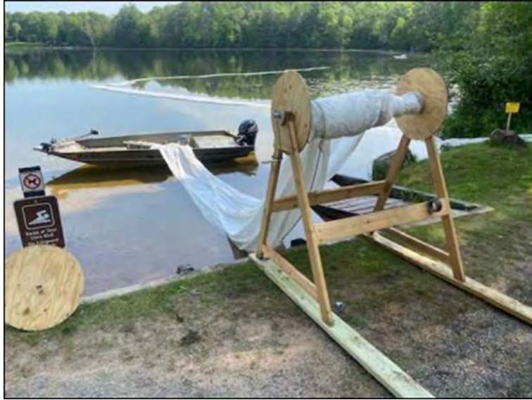
Figure 67: Limno-curtain material on a roll before installation (photo from Marinette Co. LWCD)
